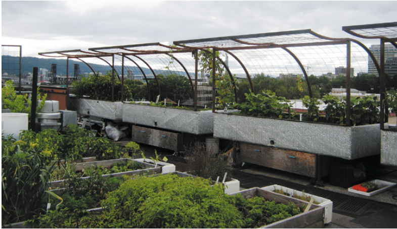
Figure 4.4 Ecoroof in Portland. (Source: Nunzia Borrelli)
