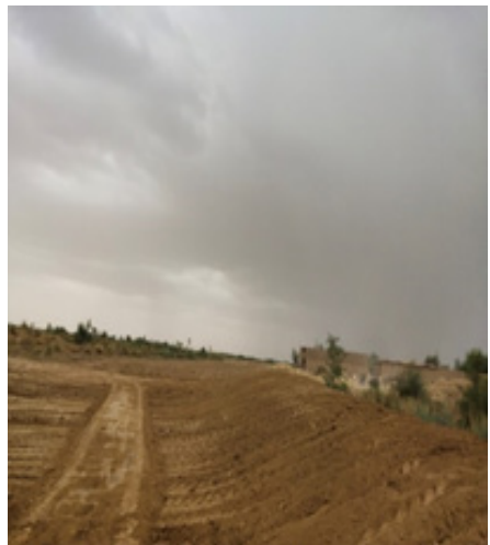
Figure 2: After the construction of Dike
