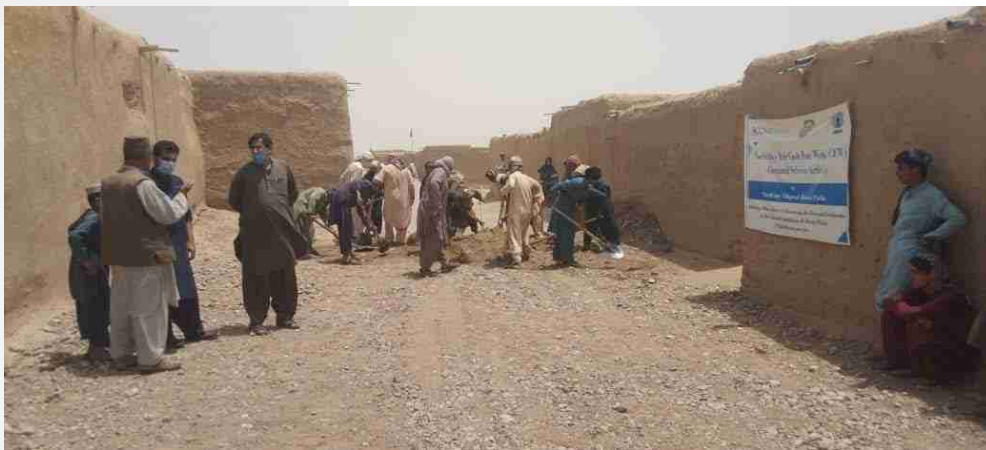
Street pavement RV Pishin
