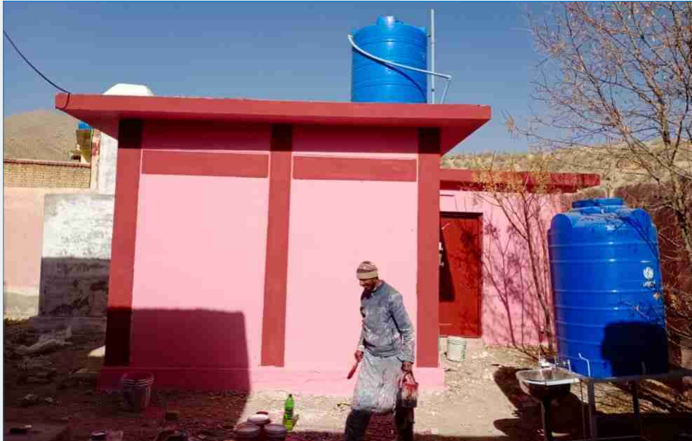
Latrine rehab BHU Hanna Urak
