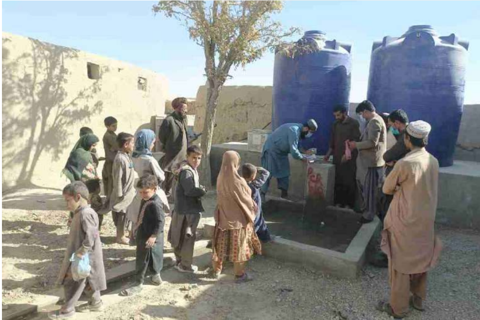
Water Tanker Installation at Loralai RV
