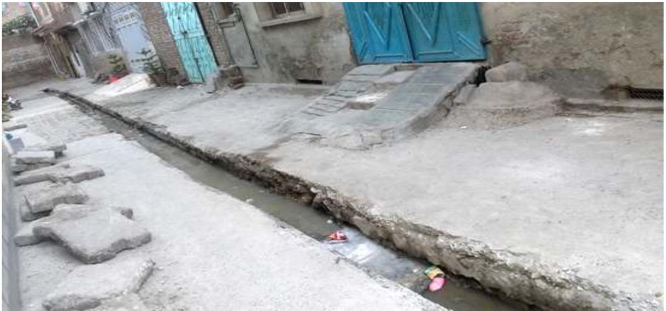
Figure: 4. vulnerable condition of the sewage system, Source: Field data, 2018
