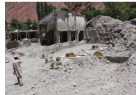
Landslides as a result of deforestation
